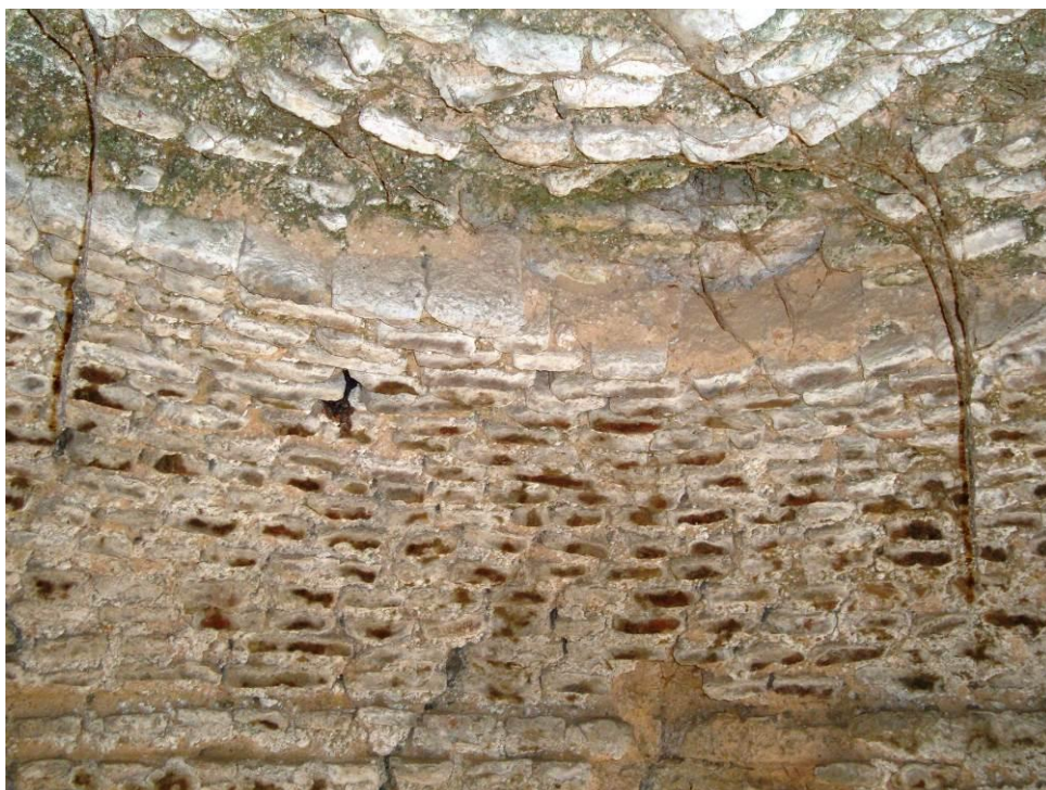
Pl. X. An inner view of Ceiling of theDome of the Chamber
